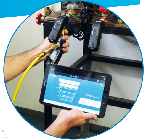
MEASURE EVACUATION WITH THE SI-RV3 VACUUM PROBE
