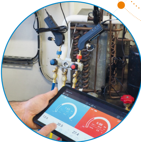
PERFORM CHECKS WITH THE SI-RM13 COMBINED MANIFOLD
