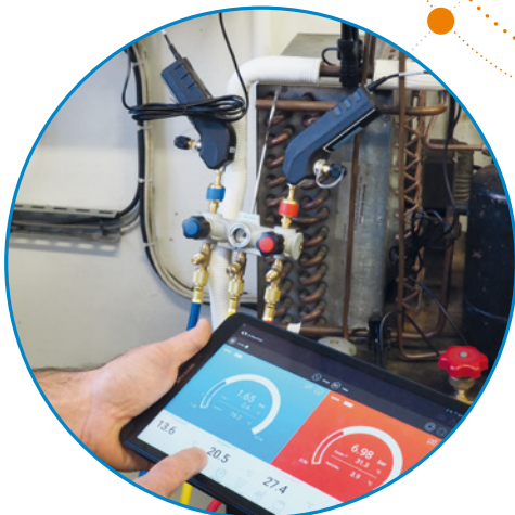
PERFORM CHECKS WITH THE SI-RM13 COMBINED MANIFOLD
